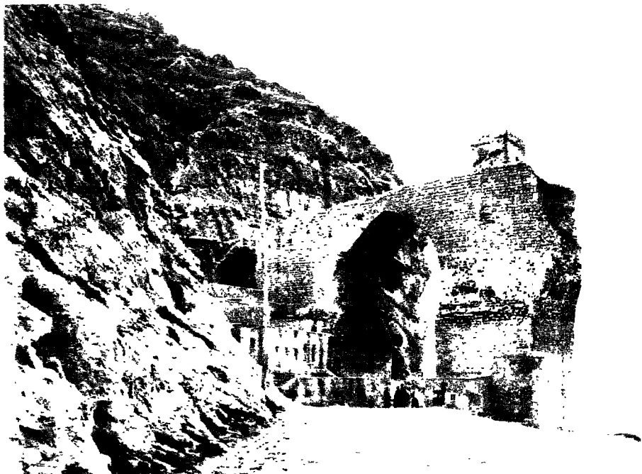
58. PIERS AND ARCH OF PUL-I-DUKHTAR BRIDGE. ON LEFT BANK OF KĀSHGĀN RIVER
